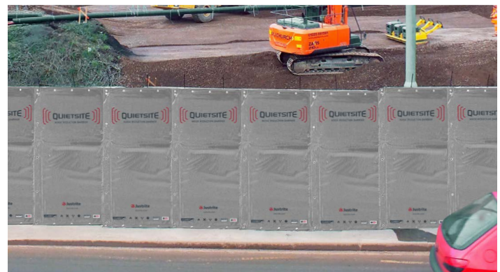
The NYC Noise Code mandates every construction site have a noise mitigation plan on location. It recognizes portable barriers with sound insulation for mitigation measures. Shown here, Justrite barriers create a sound-minimizing enclosure between a job site and a pedestrian walkway.
