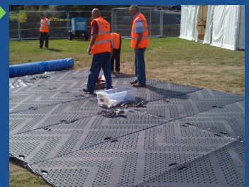
Laying double width access trackway ▶
